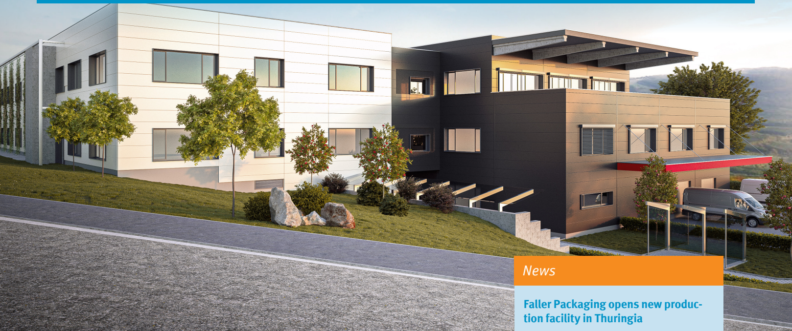
The new building of Analytik Jena in Ilmenau with a view of the Thuringian Forest. Photo: © Analytik Jena
