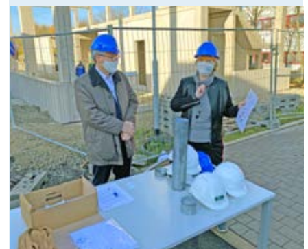
The foundation stone for the new development center is laid. Photo: Antennentechnik Bad Blankenburg GmbH
